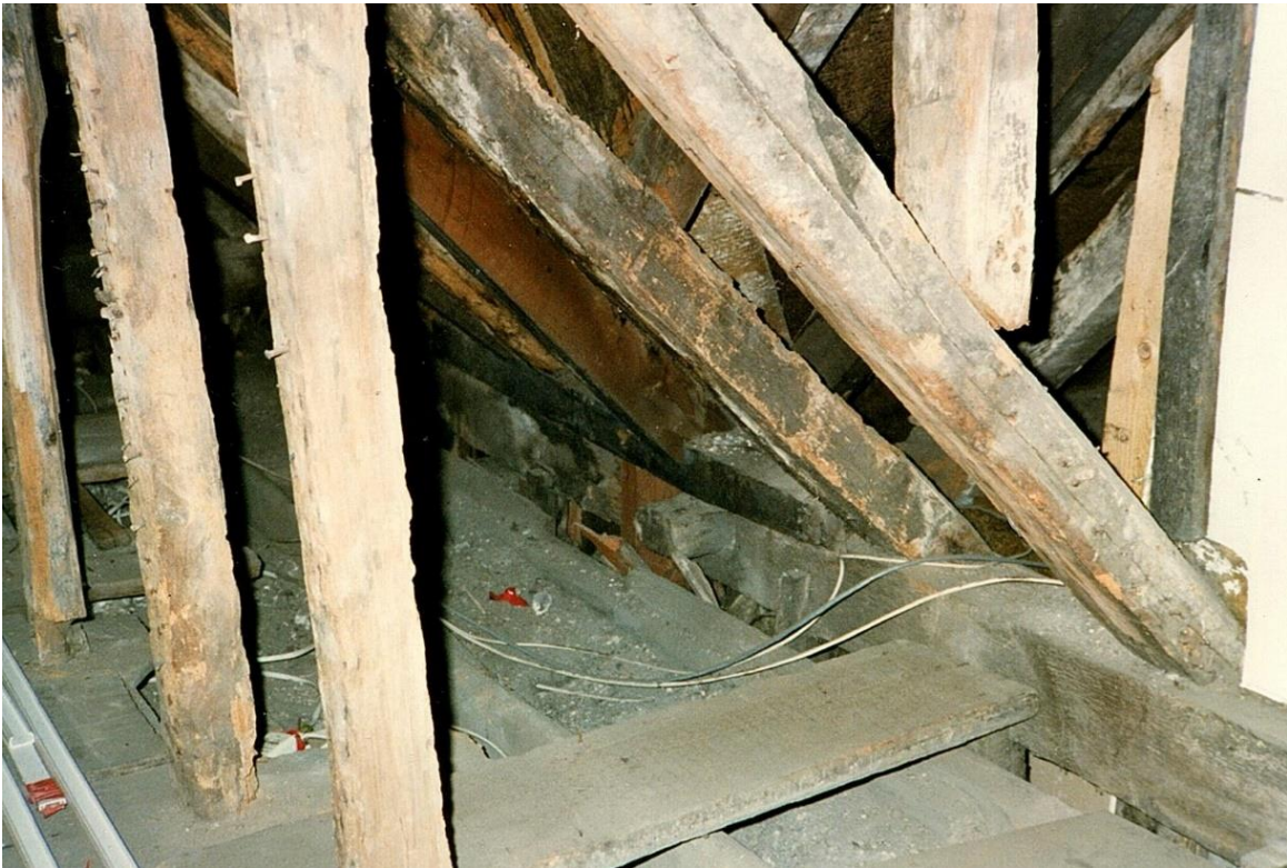
Number 1268. November 1991. East wall. Detail of sole plate and tie beam.
