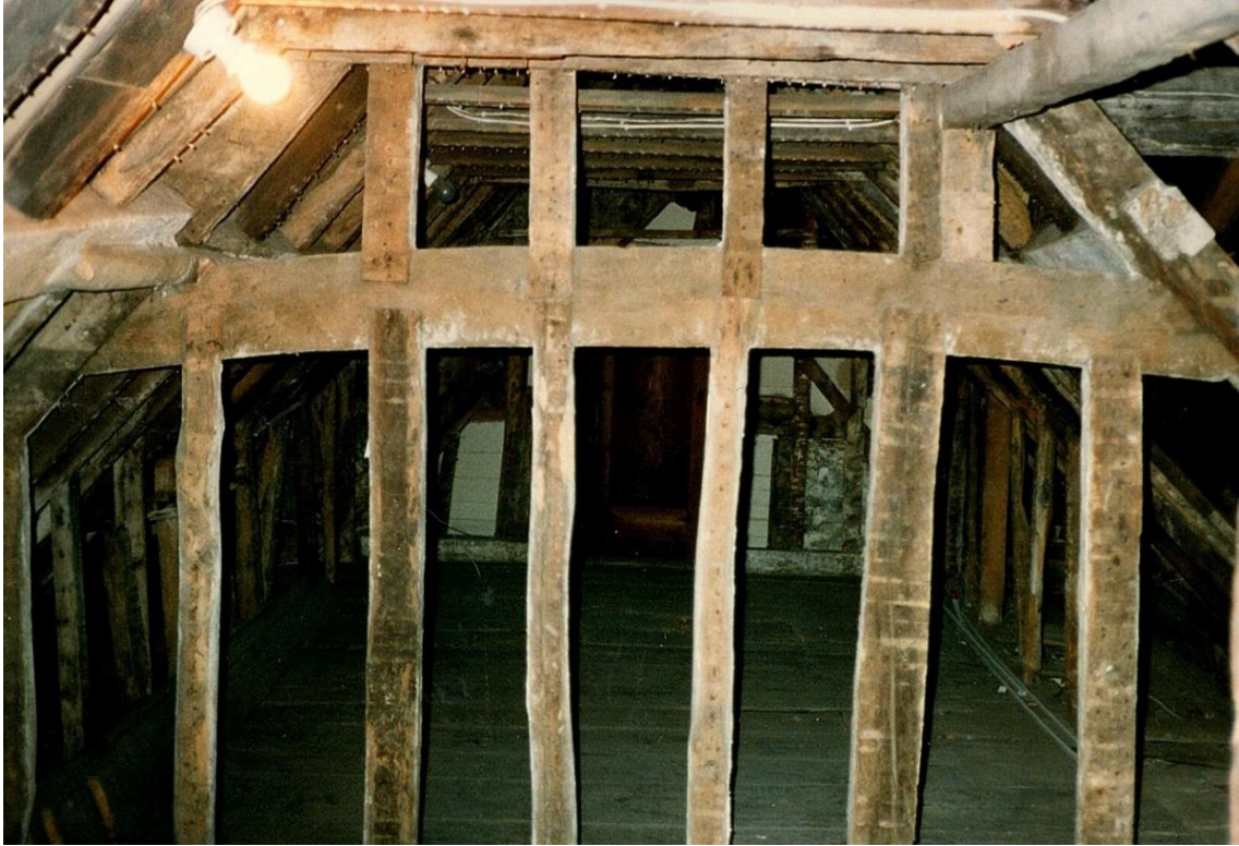
Number 1268. November 1991. Collar utilised to form later partition wall. From south.
