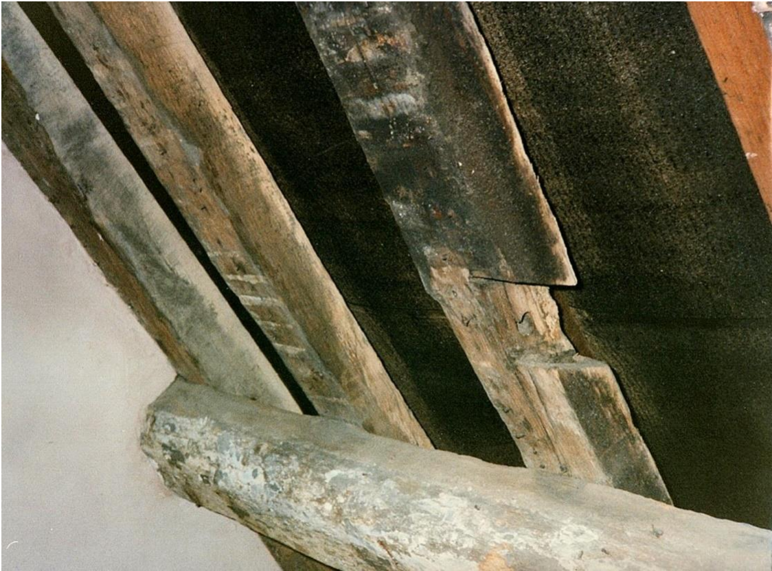
Number 1268. November 1991. Detail of apex, mortise and tenon with wooden peg.
