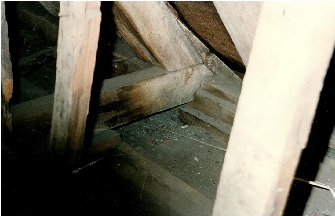
Number 1268. November 1991. West wall. Sole plate showing rafter joint.
