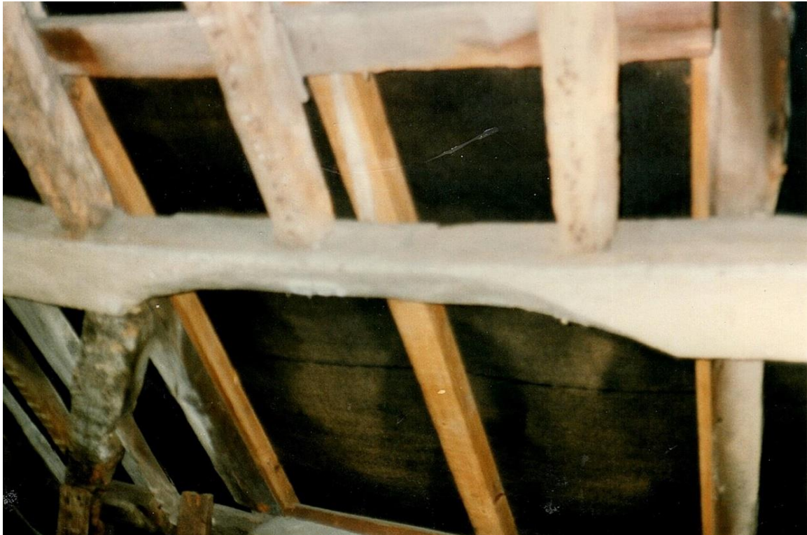
Number 1268. November 1991. Window frame now blocked off. Still visible in 1945.
