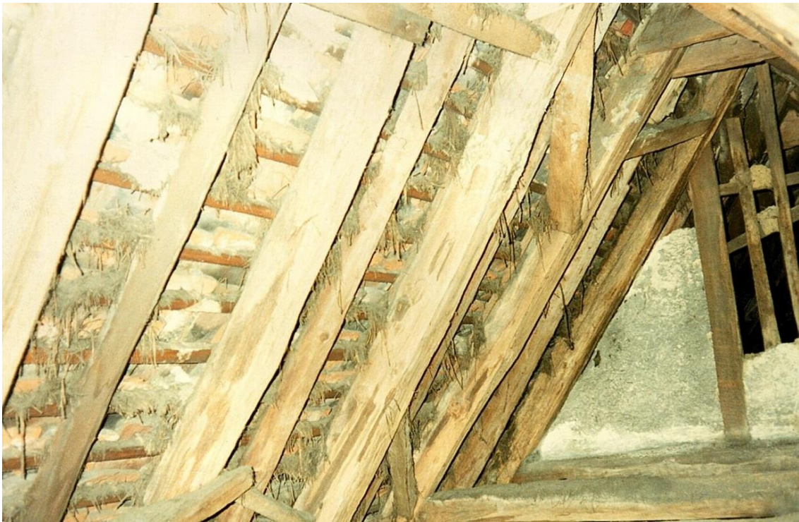
Number 1264. October 1989. Roof north side showing rafters, purlins, ceiling joists.
