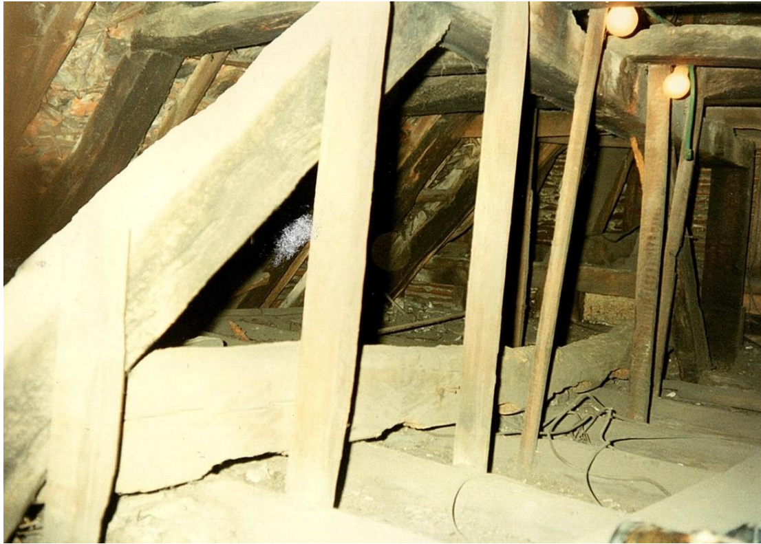
Number 1264. October 1989. Roof. Central longitudinal beam from east.
