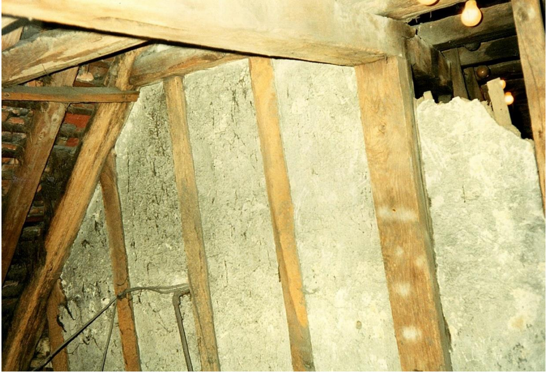
Number 1264. October 1989. Roof. Victorian lath and plaster. Victorian timber.
