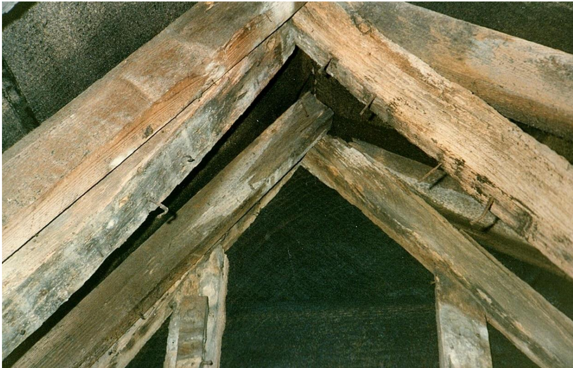
Number 1268. November 1991. Apex joint of rafters.
