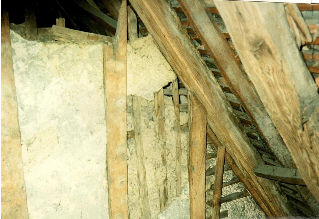
Number 1264. October 1989. Roof partition, Victorian plaster and earlier wattle and daub. Medieval rafter.
