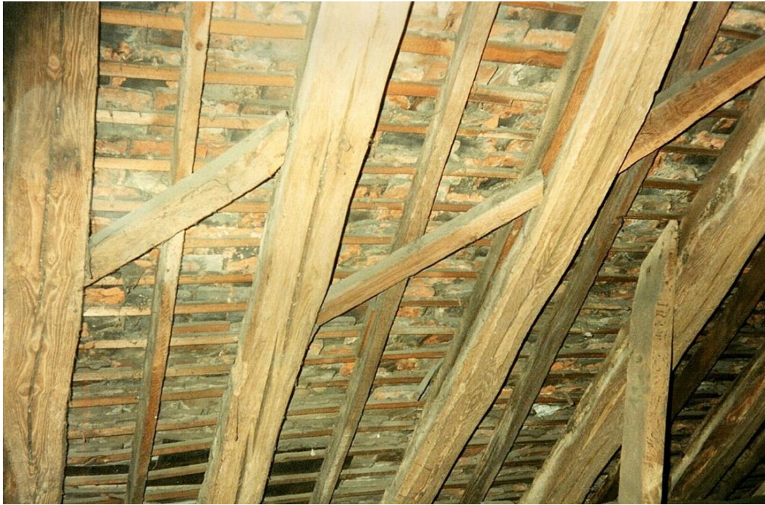
Number 1264. October 1989. Roof northside, rafters and purlins.
