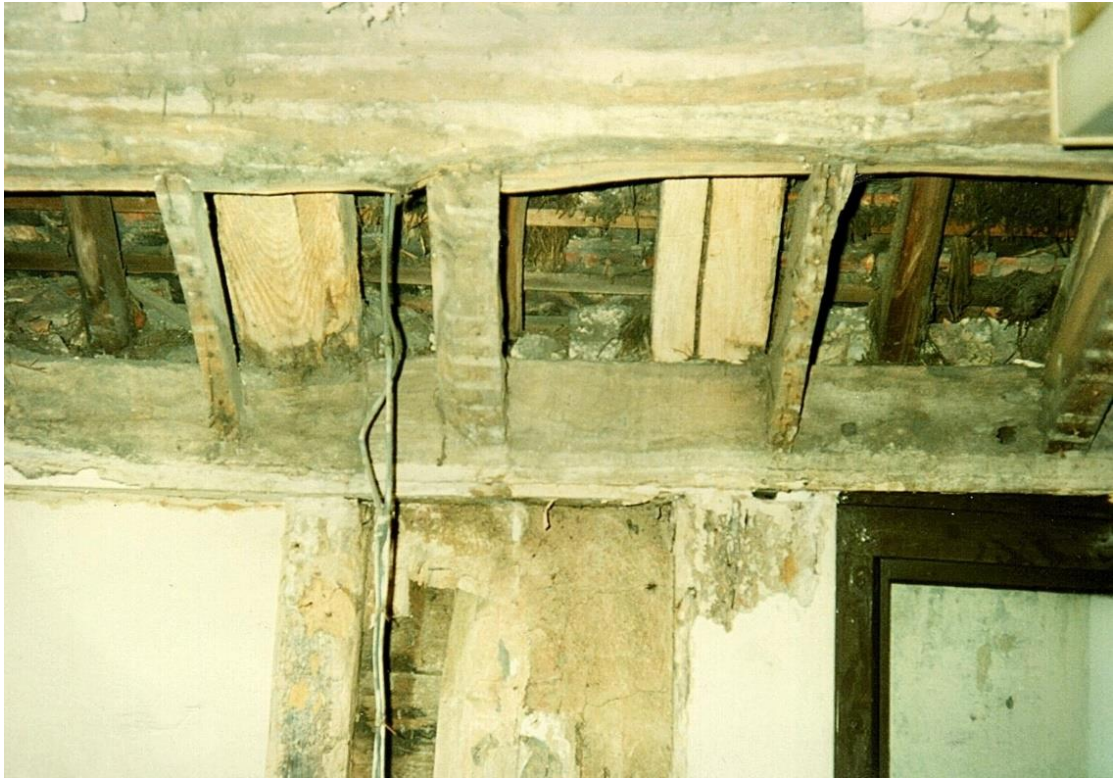
Number 1264. October 1989. Rear ground floor room. Detail of ceiling timbers.
