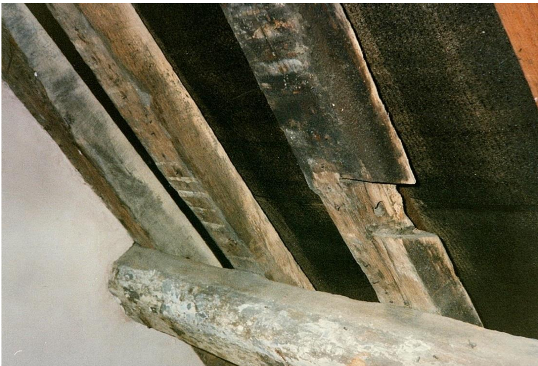
Number 1268. November 1991. Purlin – chamfered. C16?
