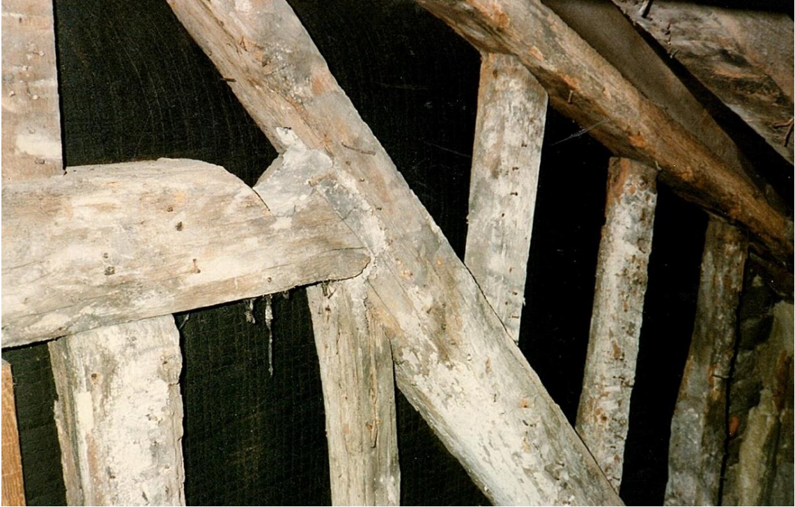
Number 1268. November 1991. Clasped purlin has been removed.
