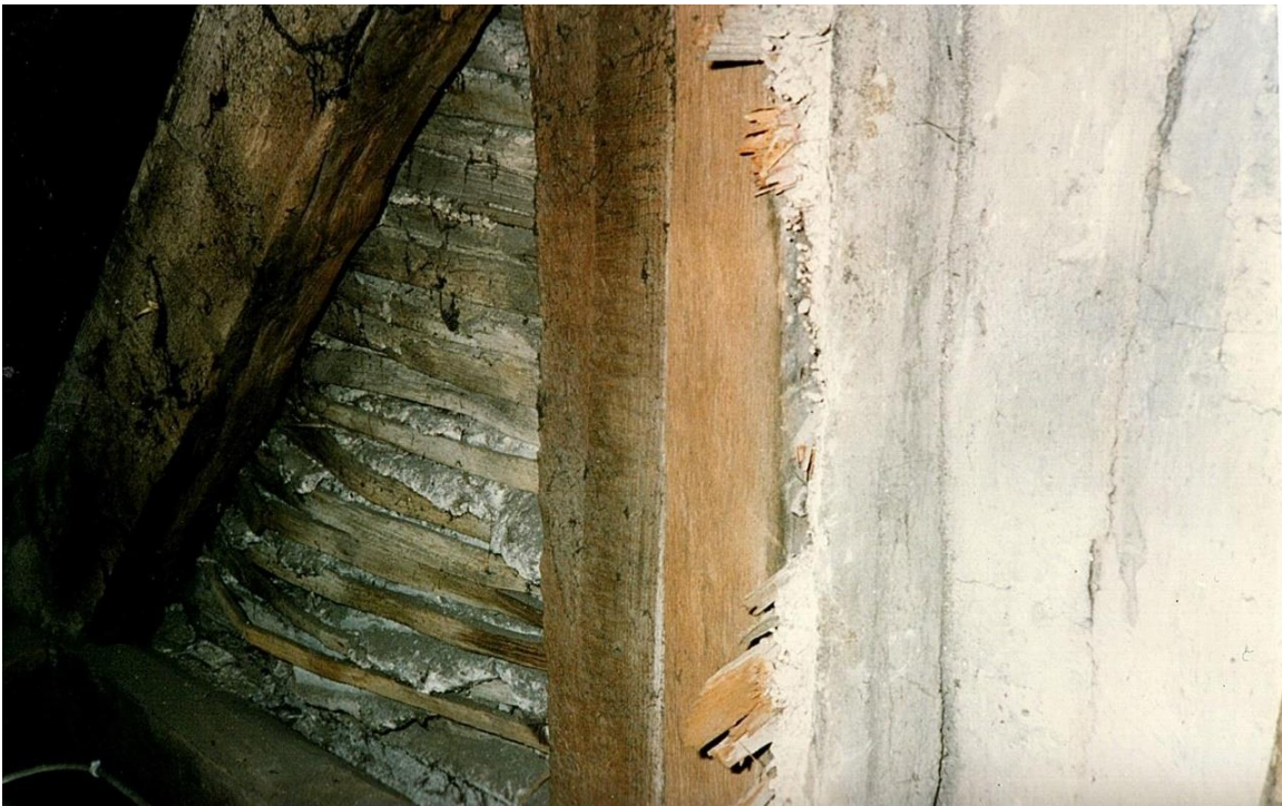
Number 1268. November 1991. Wattle and daub in S E corner of attic.
