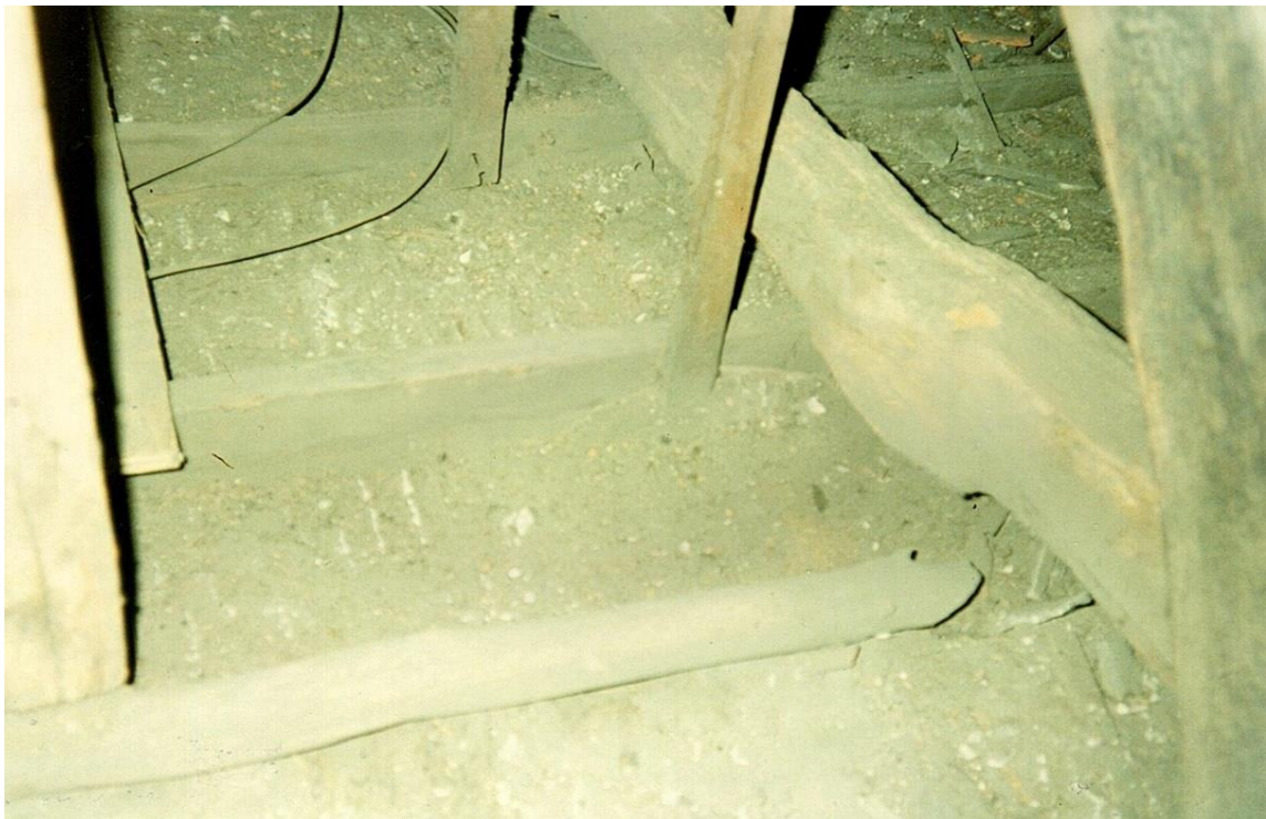
Number 1264. October 1989. Roof. Main longitudinal ceiling joists.
