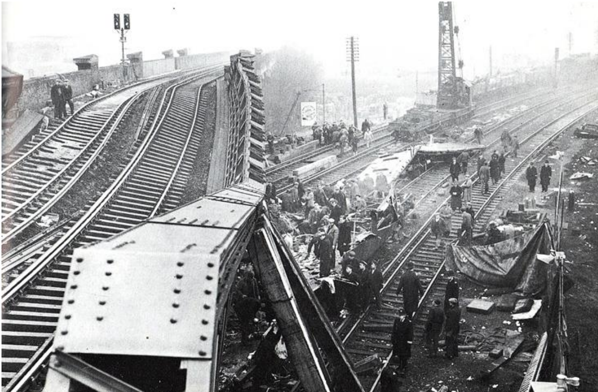
Clearing up after the Lewisham crash. The overbridge had collapsed and had to be rebuilt
