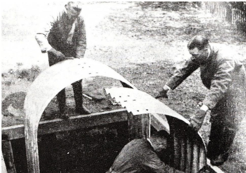
An Anderson Shelter under construction
